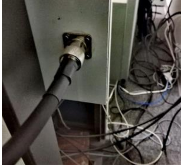
Figure 13.2: Antenna line connection
